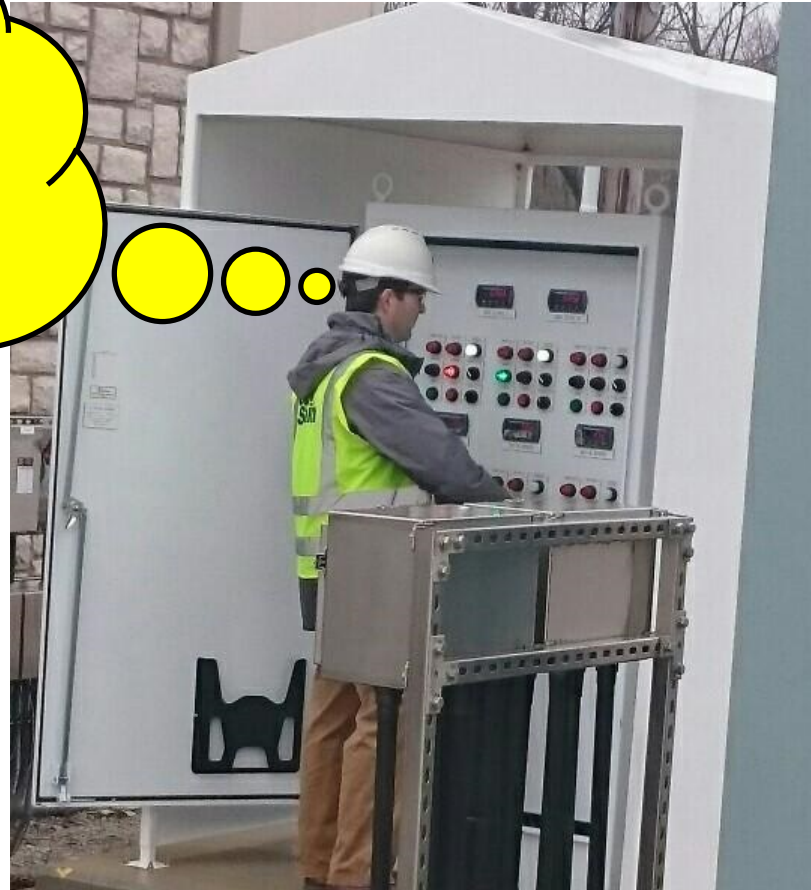
The first pump start with sewage
