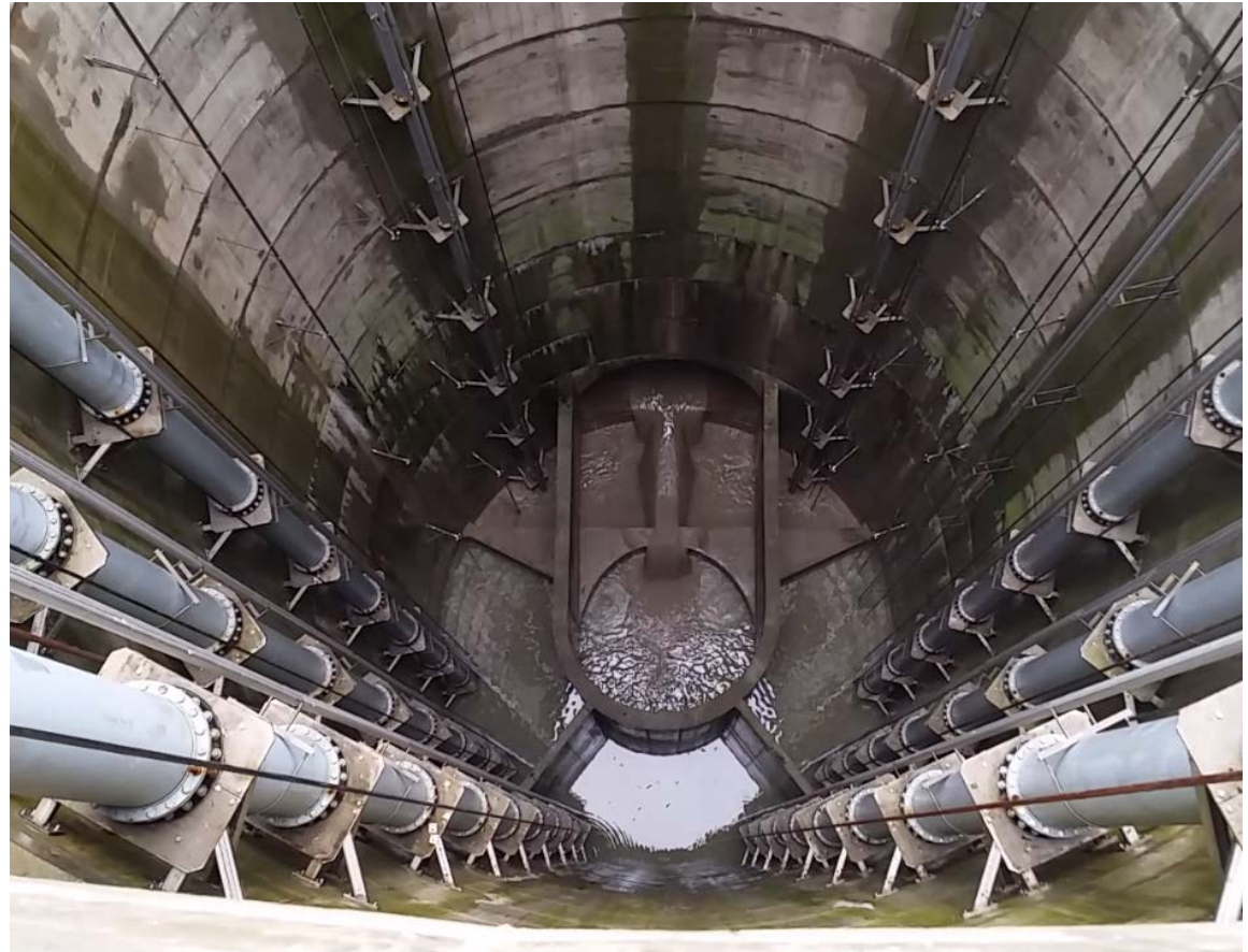
First tunnel filling test
