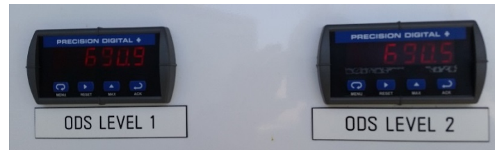
Local Control Panel
