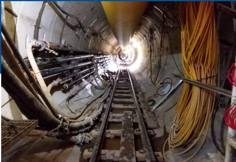
View in the tunnel with utilities and air piping shown.
