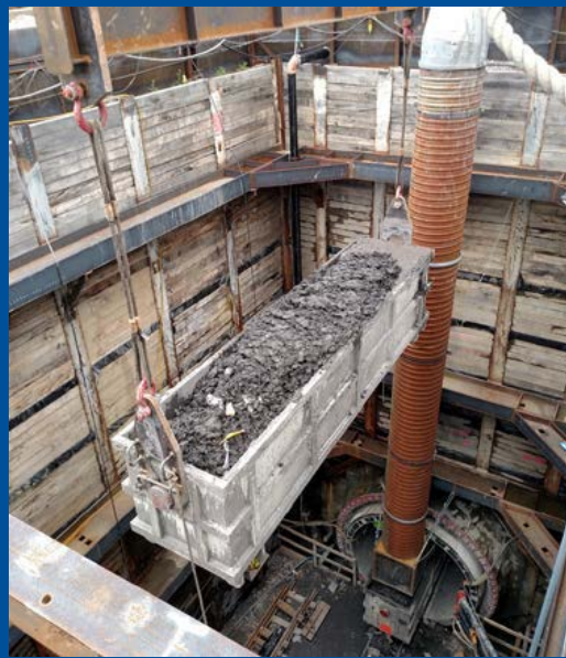
Tunnel muck being removed from Shaft 1
