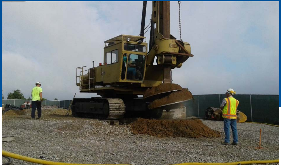
Start of drilling of MH 2B
