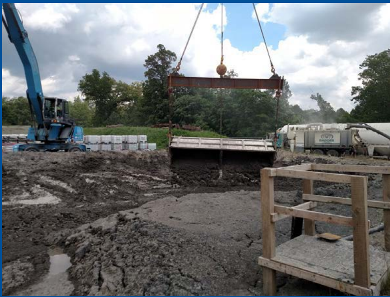
Muck being dumped in the muck pond
