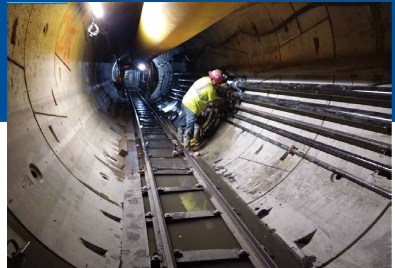
Utility Extension Work in Tunnel
