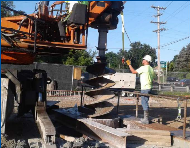
Drilling Shaft 3B.
