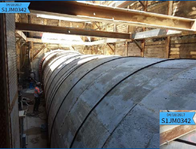
Shaft 1 with push rings installed for TBM launch
