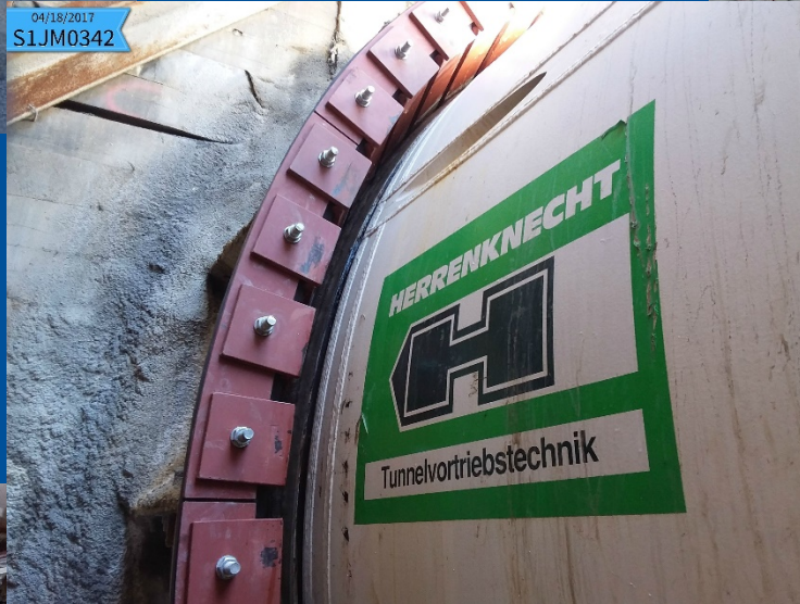
Shaft 1 with top half of push rings removed
