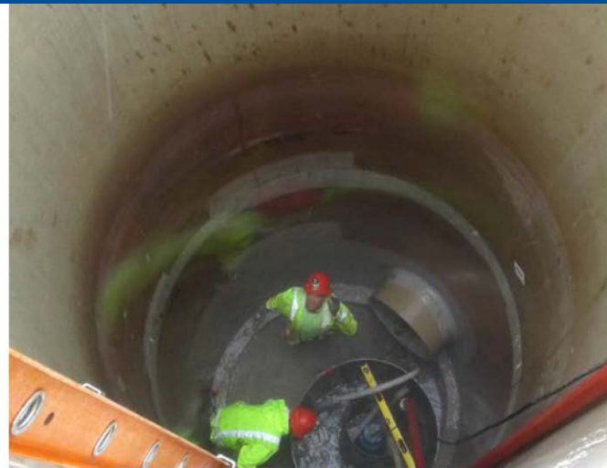
Inside of MH 3B where the connection from MH3C enters.
