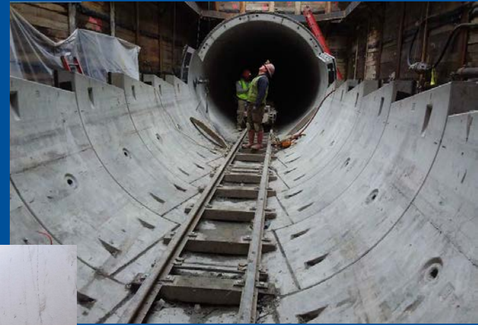
Shaft 1 with top half of push rings removed
