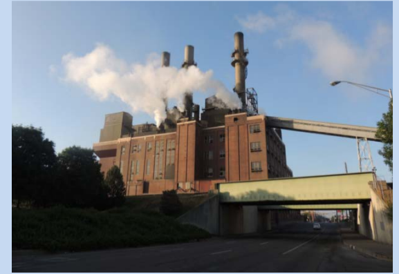
Perry K Steam Plant
