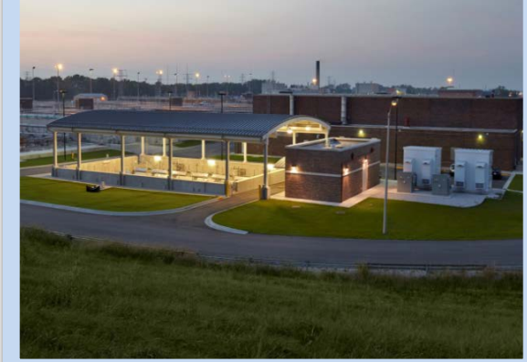
Advanced Wastewater Treatment Plants
