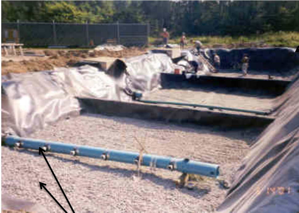
Aggregate for Underdrain and Main Air Distribution Header
