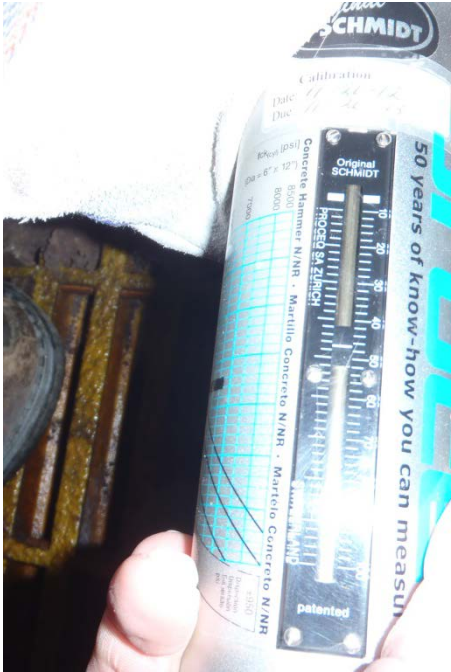
Schmidt Hammer Testing
