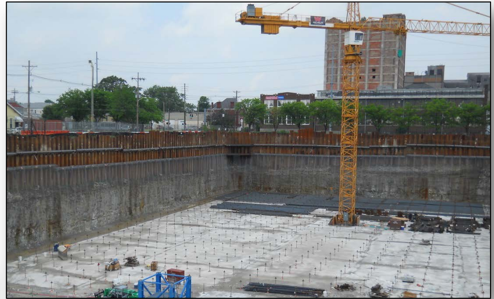
Logan St Basin Construction
