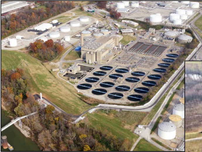
Wastewater collection and treatment
