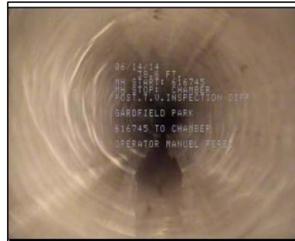
Finished CIPP liner
