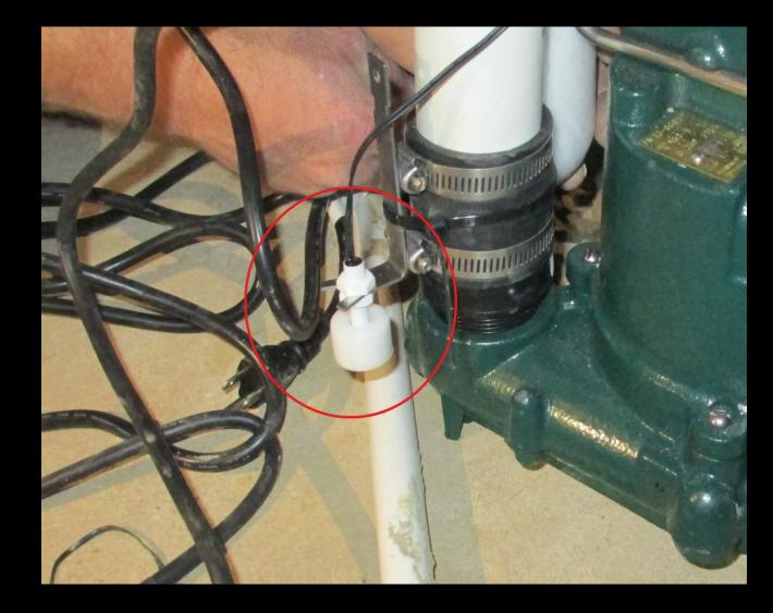
The data logger is a retired ADS Flowshark meter using the rain gauge port to count the float switch closures.
