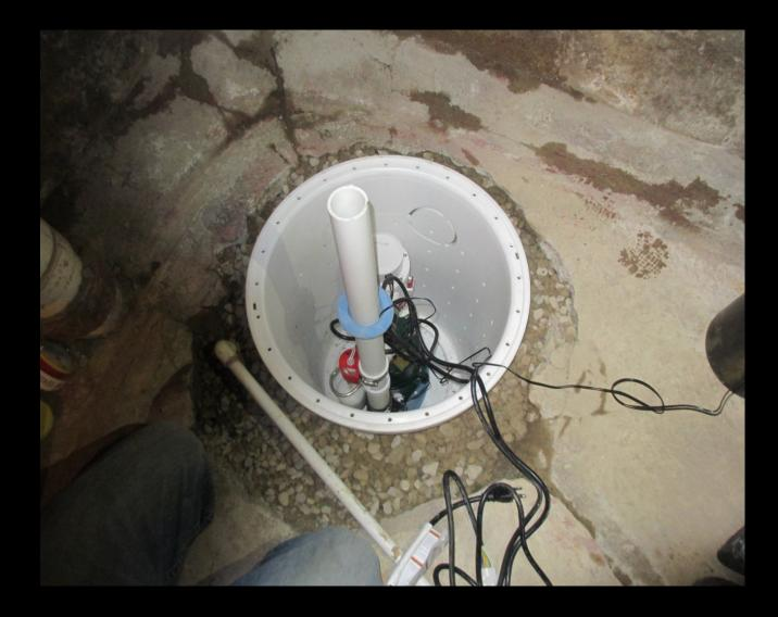
Complete install, showing discharge piping, inline ZPM water meter, backup battery, and float switch data logger.
