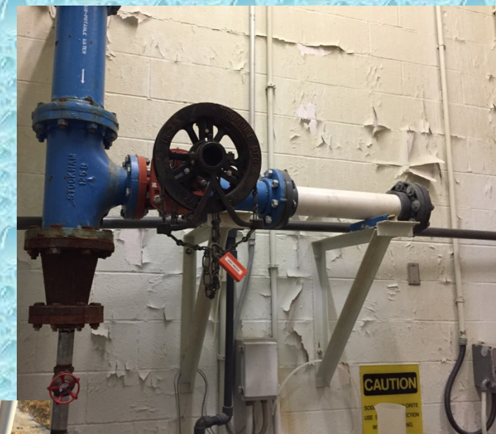
Failed Carry Water Piping
