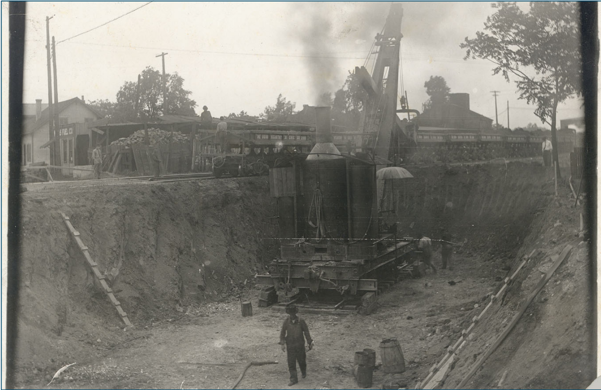
1914 Construction Photo of Lower Pogues Run Box Culvert
