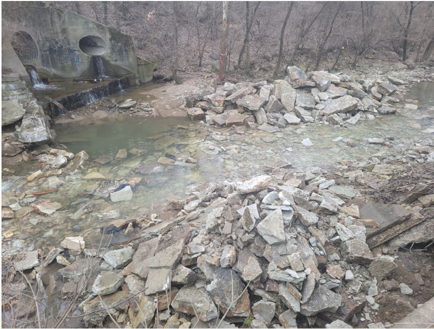
Reuse concrete slabs
